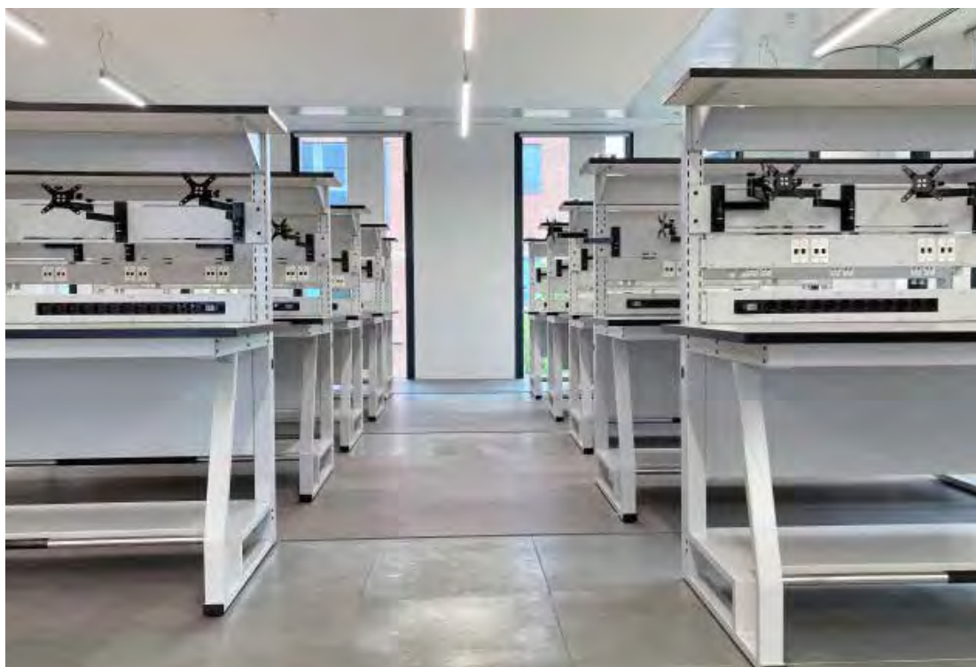
Equipped with a double 12 schuko power module and a RJ45 connection module. (fig.2)
